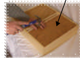
STEP 8: Tack plywood in place with four nails on the ends and three per plywood panel along the sides.
